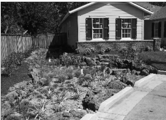
This bioretention area in a new development is an example of LID. Photo courtesy of Tom Dalziel, Contra Costa Clean Water Program
