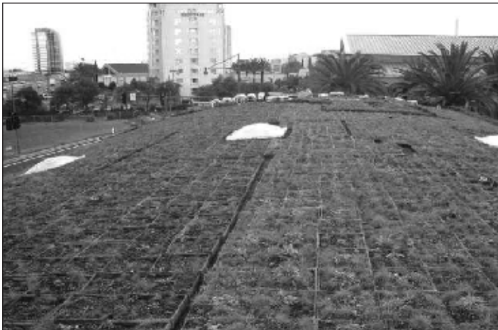
This green roof installation on a commercial building is an example of LID. Photo courtesy of Peter Schultze-Allen, City of Emeryville, CA
