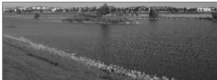
This detention basin serving a residential development is an example of a treatment control BMP. Photo courtesy of Donna Bodine
