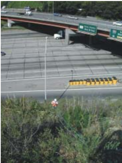
Third Street Light Rail is becoming a reality, connecting Bay View/Hunters Point with Mission Bay and downtown. This is the Third Street/U.S. 101 bridge that will be reconstructed to accommodate the light rail.
